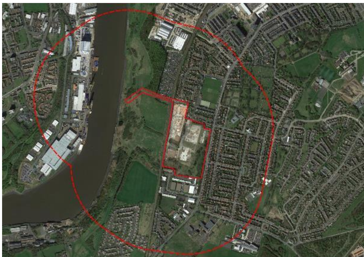
FIGURE 5: SITE AND SETTING (Reproduced under licence from Google Earth Pro.)
